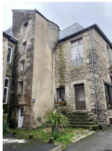
Élévation nord Phot. Baptiste Oligo IVR53_20265610182NUCA
