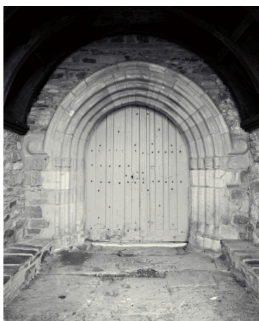
Porte sud Phot. Guy Artur, Phot. Norbert Lambart IVR53_19943501759X
