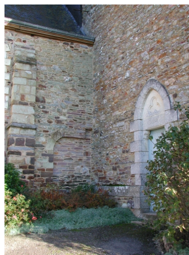
Raccord nef et transept Phot. Claude Quillivic IVR53_20003510640NUCA
