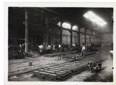
Usine Chaffoteaux-et-Maury Phot. Raphaël BINET IVR53_20262210060NUCB
