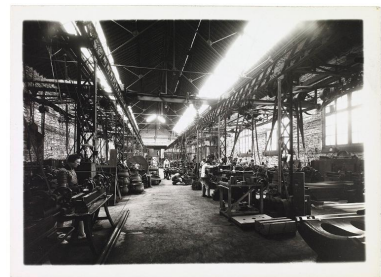
Usine Chaffoteaux-et-Maury Phot. Raphaël BINET IVR53_20262210059NUCB
