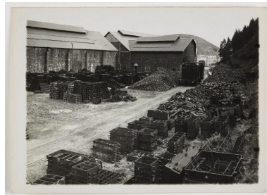
Usine Chaffoteaux-et-Maury Phot. Raphaël BINET IVR53_20262210058NUCB
