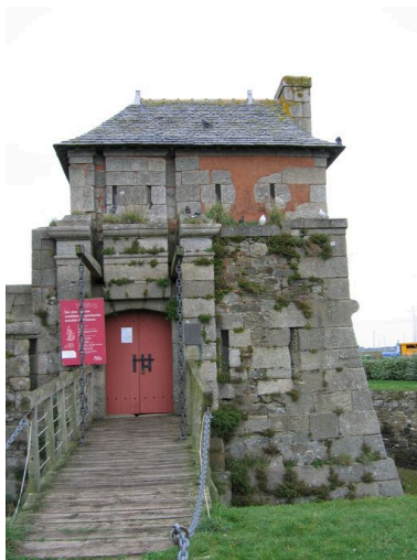
Pont-levis Phot. Guillaume Marie IVR53_20062908497NUCA
