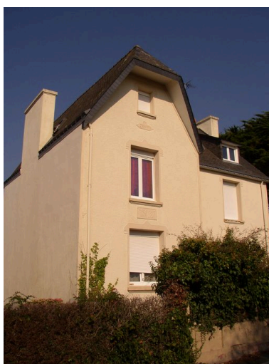
Villa Ty Jeannic Phot. Johan Vincent IVR53_20062908675NUCA
