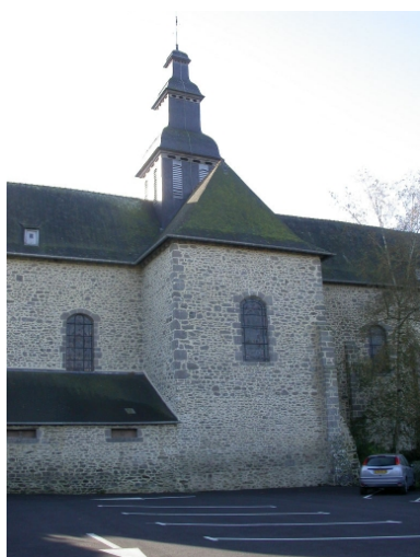
Vue nord Phot. Sabrina Dalibard IVR53_20063513955NUCA
