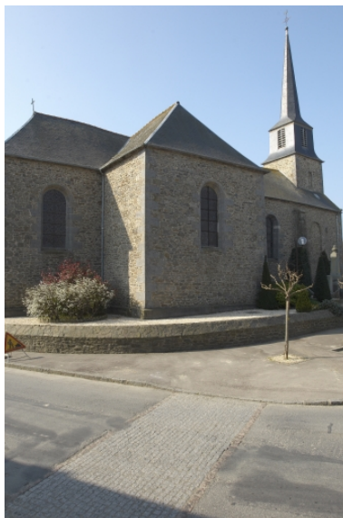
Elévation nord Phot. Norbert Lambart IVR53_20073500515NUCA
