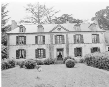
Logis, élévation nord. Phot. Guy Artur, Phot. Norbert Lambart IVR53_19895600413X
