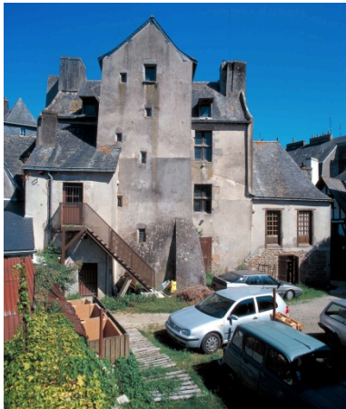
Elévation ouest Phot. Bernard Bègne IVR53_20012900059XA
