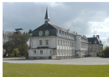
L'établissement scolaire Phot. Guy Artur, Phot. Norbert Lambart IVR53_20033500668NUCA
