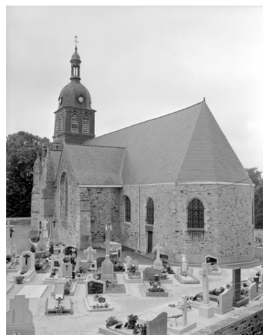
Elevation sud-est Phot. Guy Artur, Phot. Norbert Lambart IVR53_19943501506X
