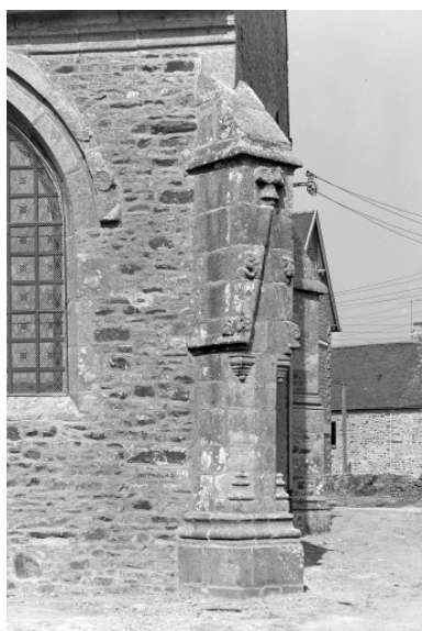
Façade sud, contrefort. Phot. Guy Artur IVR53_19723500248V
