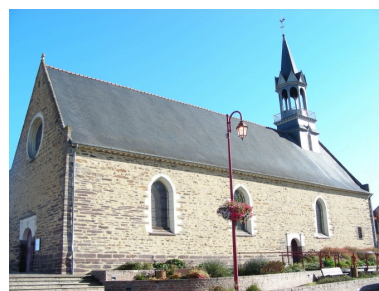
Vue sud Phot. Sabrina Dalibard IVR53_20073508607NUCA
