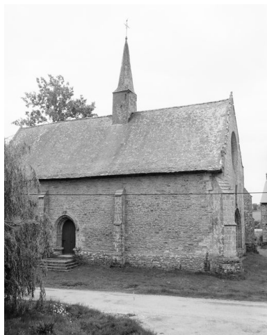
Elévation nord Phot. Guy Artur, Phot. Norbert Lambart IVR53_19915600554X
