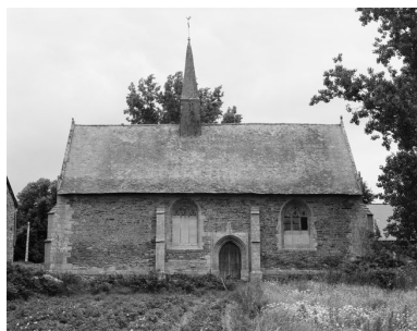
Elévation sud Phot. Guy Artur, Phot. Norbert Lambart IVR53_19915600551X
