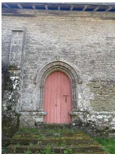
Porte, élévation nord Phot. Baptiste Oligo IVR53_20265610604NUCA
