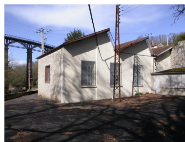
La "salle de relayage", façade sud. Phot. Marina Gasnier IVR53_20042203089NUCA
