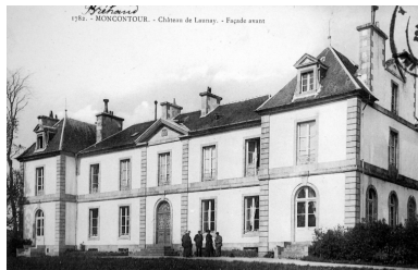
Elévation antérieure Phot. Elise Lauranceau IVR53_20042209041NUCB
