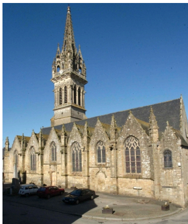
Façade sud Phot. Guy Artur, Phot. Norbert Lambart IVR53_20033517886NUCA
