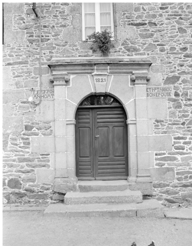
Porte sud Phot. Guy Artur IVR53_19752200233X
