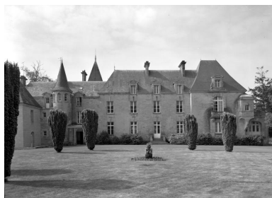
Façade antérieure Phot. Guy Artur, Phot. Norbert Lambart IVR53_19885601471V
