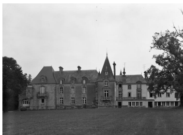
Façade postérieure Phot. Guy Artur, Phot. Norbert Lambart IVR53_19885601466V
