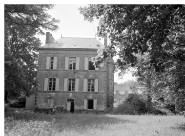
Elévation postérieure. Phot. Norbert Lambart IVR53_19815600466X
