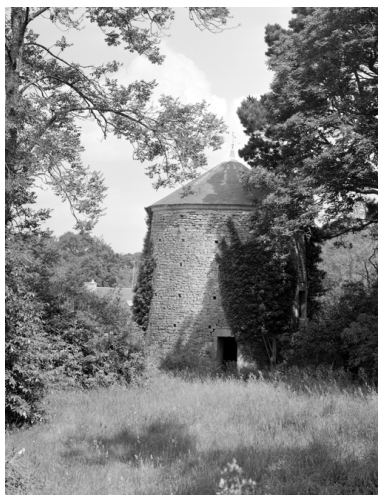
Colombier, vue sud. Phot. Norbert Lambart IVR53_19815600465X
