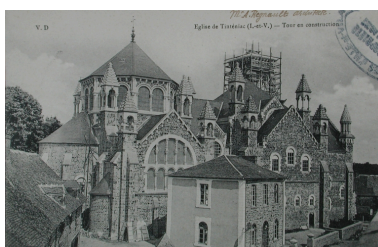
Construction du clocher Phot. Elise Lauranceau IVR53_20063512073NUCB
