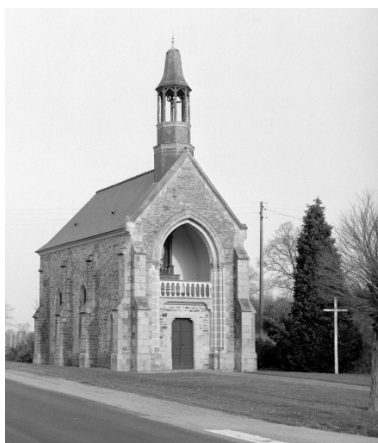
Elévation nord-ouest. Phot. Guy Artur, Phot. Norbert Lambart IVR53_19933500121X
