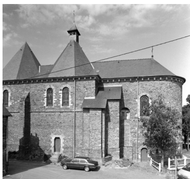
Elévation Est, partie nord Phot. Guy Artur, Phot. Norbert Lambart IVR53_19943501765X
