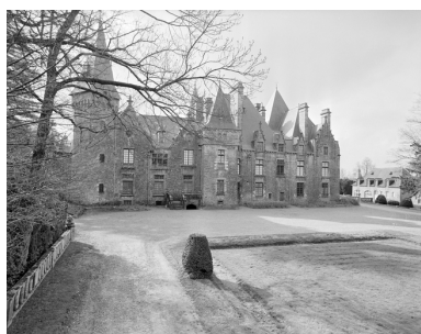
Elévation nord. Phot. Guy Artur, Phot. Norbert Lambart IVR53_19963500820X
