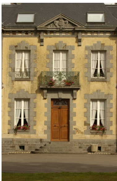
La travée centrale Phot. Norbert Lambart IVR53_20053502663NUCA
