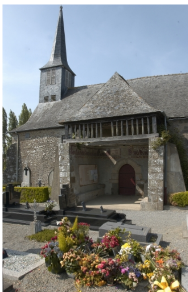
Porche sud Phot. Norbert Lambart IVR53_20043500882NUCA
