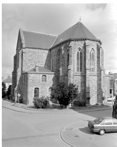
Elévation sud-est Phot. Guy Artur, Phot. Norbert Lambart IVR53_19943501323X
