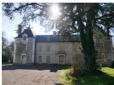
Façade principale Phot. Tiphaine Berger IVR53_20193505439NUCA
