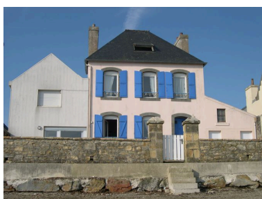
Maison Tertu Phot. Clotilde Buhot IVR53_20062908580NUCA
