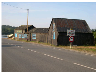
Chantier Stipon Phot. Clotilde Buhot IVR53_20062908517NUCA
