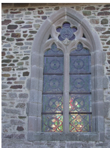
Nef, mur nord, (baie 7) Phot. Marie-Dominique Menant IVR53_20073506468NUCA
