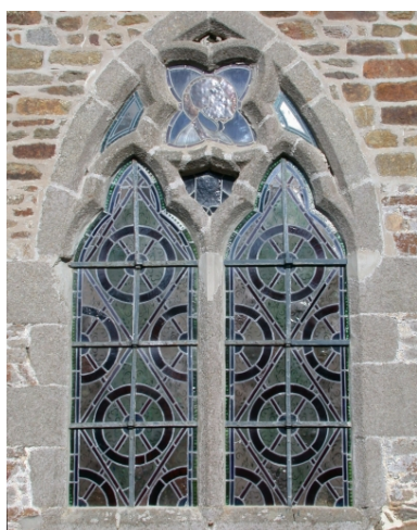
Nef, mur sud, (baie 12) Phot. Marie-Dominique Menant IVR53_20073506472NUCA
