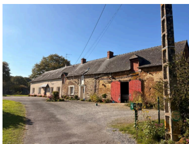
493 Ventrillon Phot. Kawrentin Pichot IVR53_20263510402NUCA
