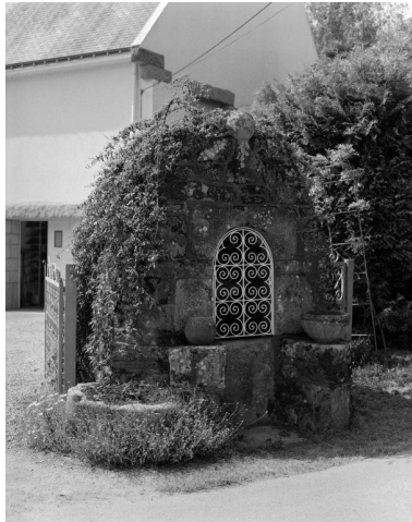
Puits. Phot. Guy Artur, Phot. Norbert Lambart IVR53_19925600918X
