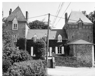
Elévation sud-ouest. Phot. Guy Artur, Phot. Norbert Lambart IVR53_19925600927X
