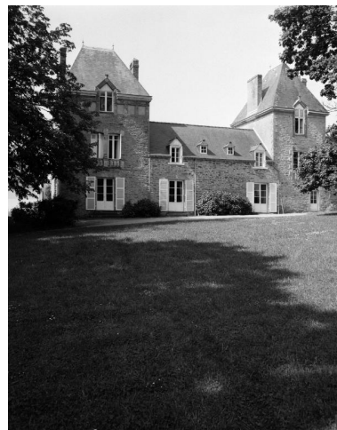
Elévation nord-est. Phot. Guy Artur, Phot. Norbert Lambart IVR53_19925600919X
