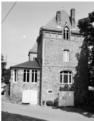
Elévation sud-est. Phot. Guy Artur, Phot. Norbert Lambart IVR53_19925600921X
