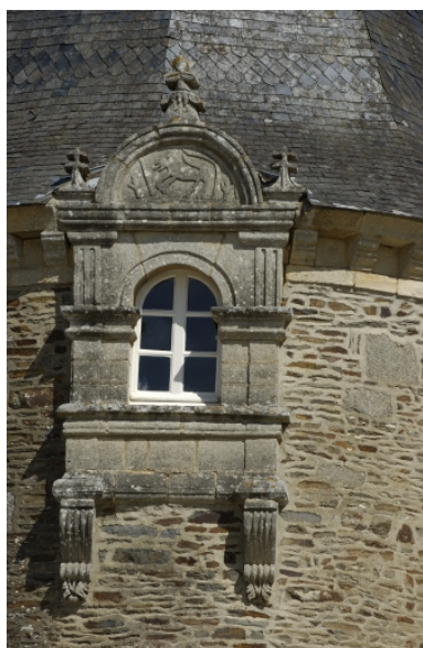
Lucarne Phot. Norbert Lambart IVR53_20063501428NUCA
