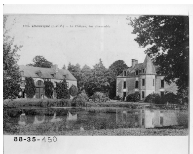
Vue de situation Phot. Guy Artur, Phot. Norbert Lambart IVR53_19883500150X
