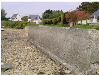
Digue du front de mer de Rostellec Phot. Clotilde Buhot IVR53_20062908536NUCA
