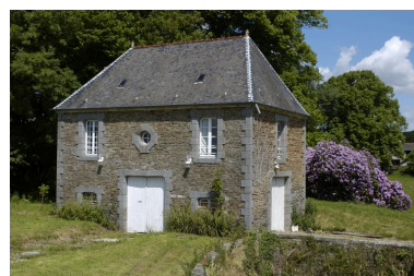
Pavillon Phot. Norbert Lambart IVR53_20063501171NUCA
