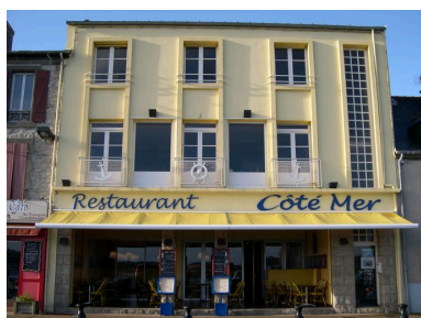
Elevation antérieure du restaurant Phot. Guillaume Marie IVR53_20062908481NUCA
