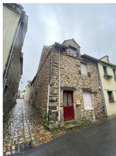
Façade nord Phot. Baptiste Oligo IVR53_20265610636NUCA
