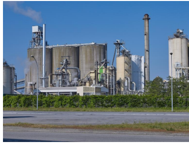
Usine de trituration Phot. Bernard Bègne IVR53_20232900391NUCA
