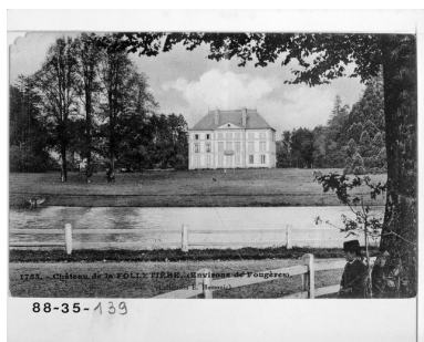
Vue de situation Phot. Guy Artur, Phot. Norbert Lambart IVR53_19883500139X
