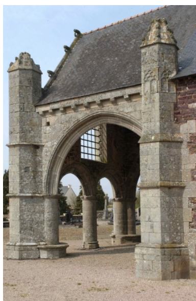
Porche, élévation sud Phot. Norbert Lambart IVR53_20033501053NUCA
