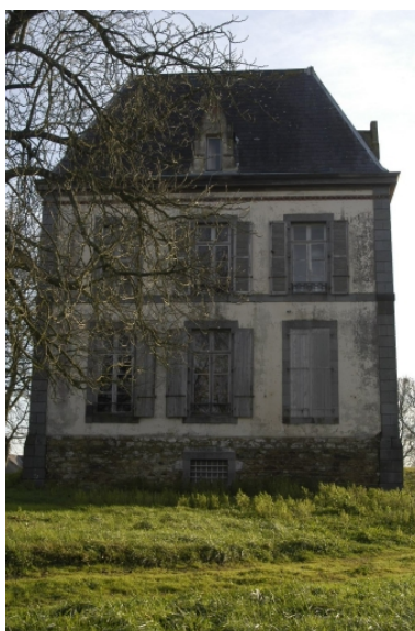
Pignon ouest Phot. Sabrina Dalibard IVR53_20063514278NUCA
