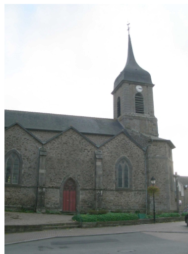
Façade nord Phot. Sabrina Dalibard IVR53_20063512583NUCA
