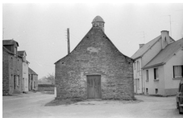
Elévation sud Phot. Berthou Marie, Phot. Catherine Toscer IVR53_19765605996Z
