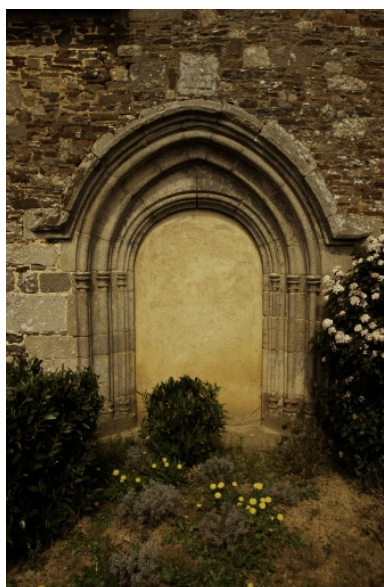
Porte sud Phot. Norbert Lambart IVR53_20063500667NUCA
