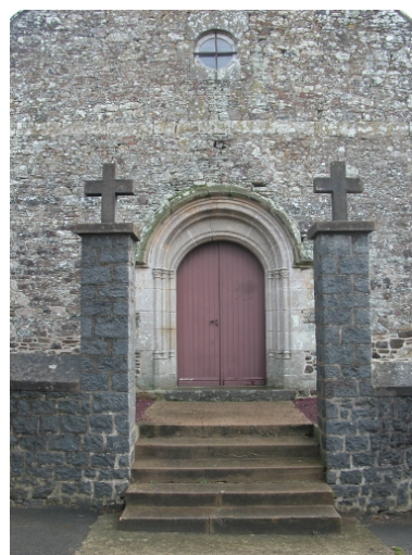
Porte ouest Phot. Claude Quillivic IVR53_20063509915NUCA
