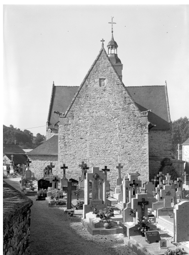
Elévation est. Phot. Guy Artur, Phot. Norbert Lambart IVR53_19843500357V
