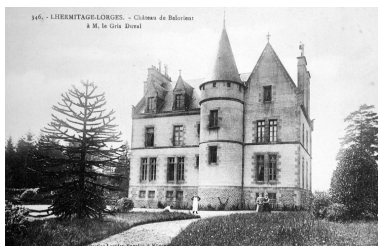
Elévations sud Phot. Elise Lauranceau IVR53_20042208997NUCB
