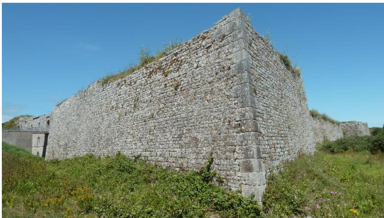
Hoedic, fort central, bastion.
