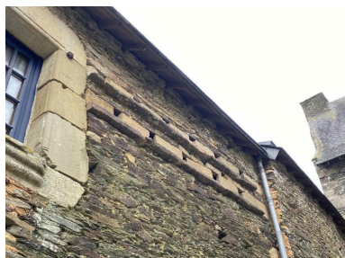
Trous de boulins, aile nord Phot. Baptiste Oligo IVR53_20265610204NUCA
