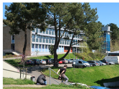
Externat D, façade sud. Phot. Thierry Goyet IVR53_20183506346NUCA
